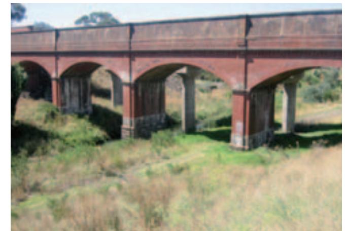
Figure 63: Historic Western Outfall Sewer Bridge (Future Site of Federation Trail)
