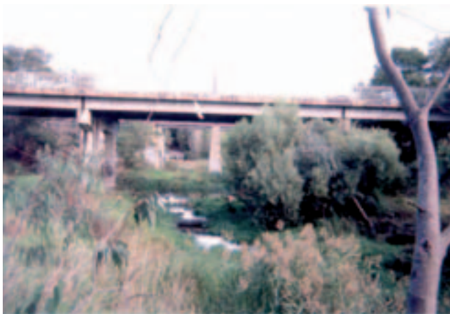
Figure 61: Forrest Street Bridge over Kororoit Creek in Sunshine West
